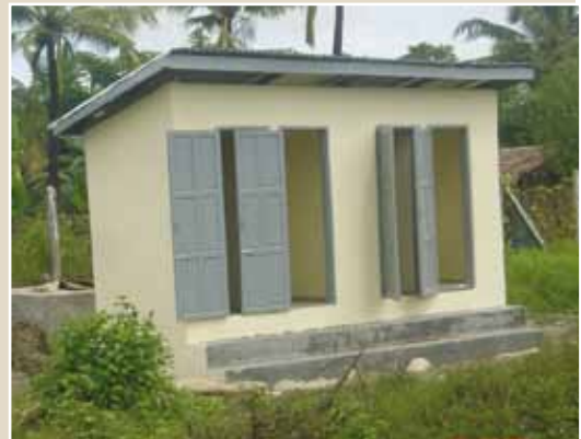
▲ Better school hygiene: one of 60 new latrines.
