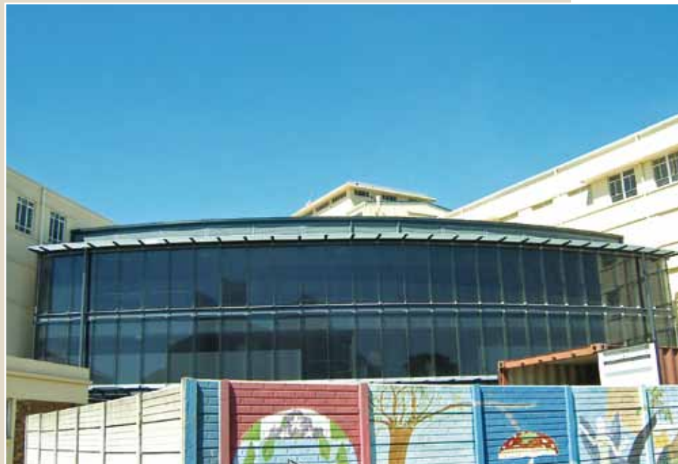
▲ The new building with the operating theater funded by Global Care.
